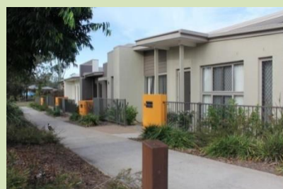
(Fitzgibbon) Front - adjoining park
