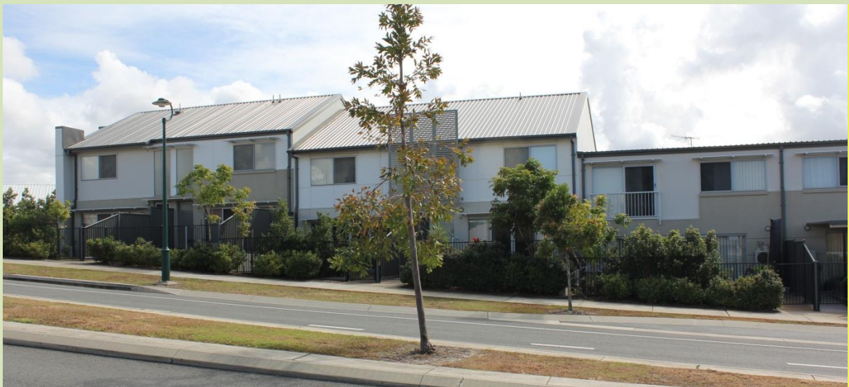
(North Lakes) Stepped terrace housing
