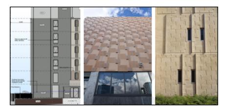
b. West facing glazing requires additional screening (bi-directional vertical screening will be most effective). EF-01 finish requires additional texture, 3d articulation and/or tonal variation as per the examples below. Darker tones to the west are discouraged due to thermal load.
